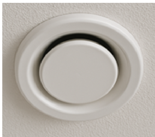
Exhaust air vent in the ceiling
